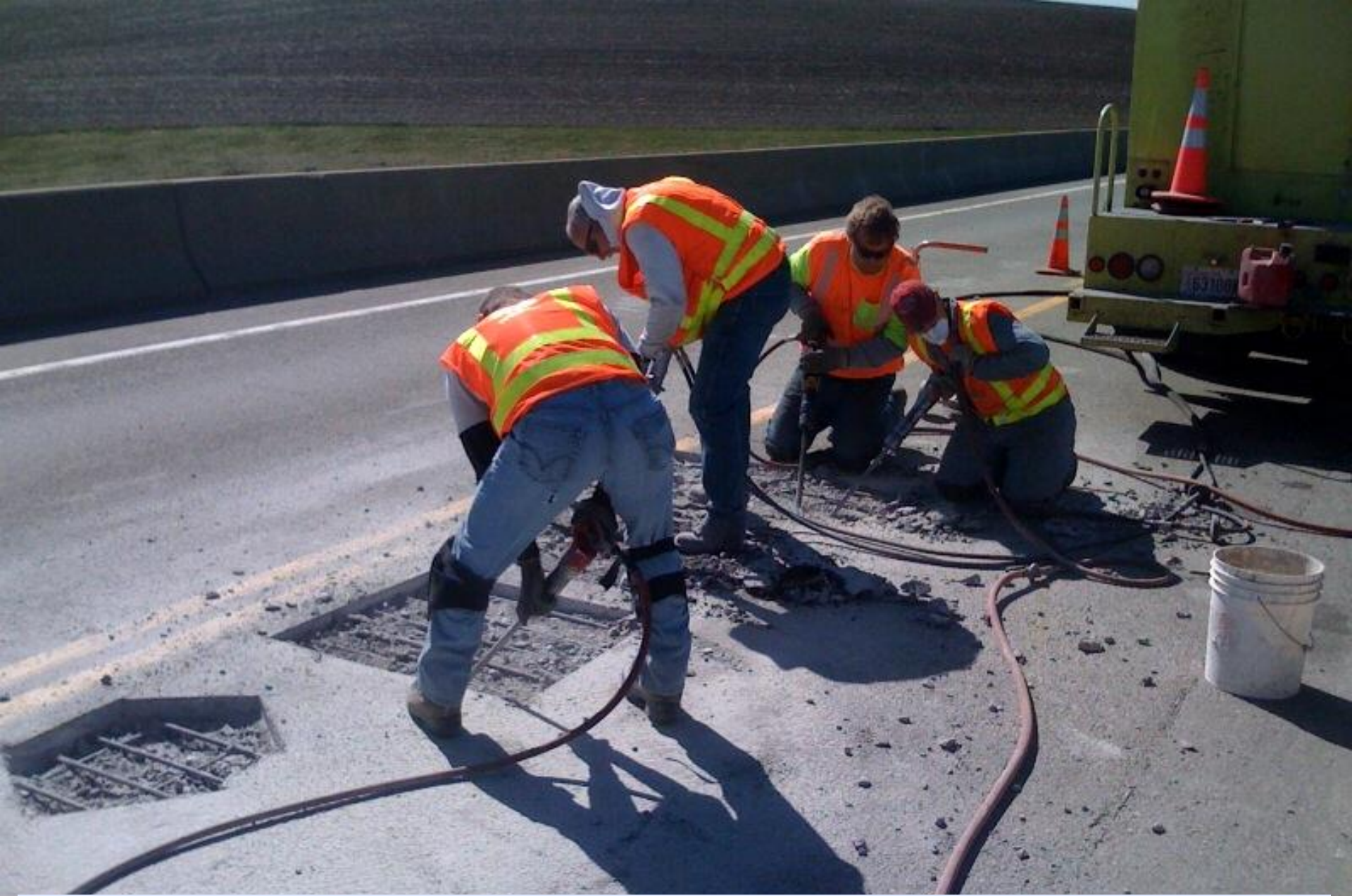
Bridge Deck Repair by WSDOT Maintenance Forces
