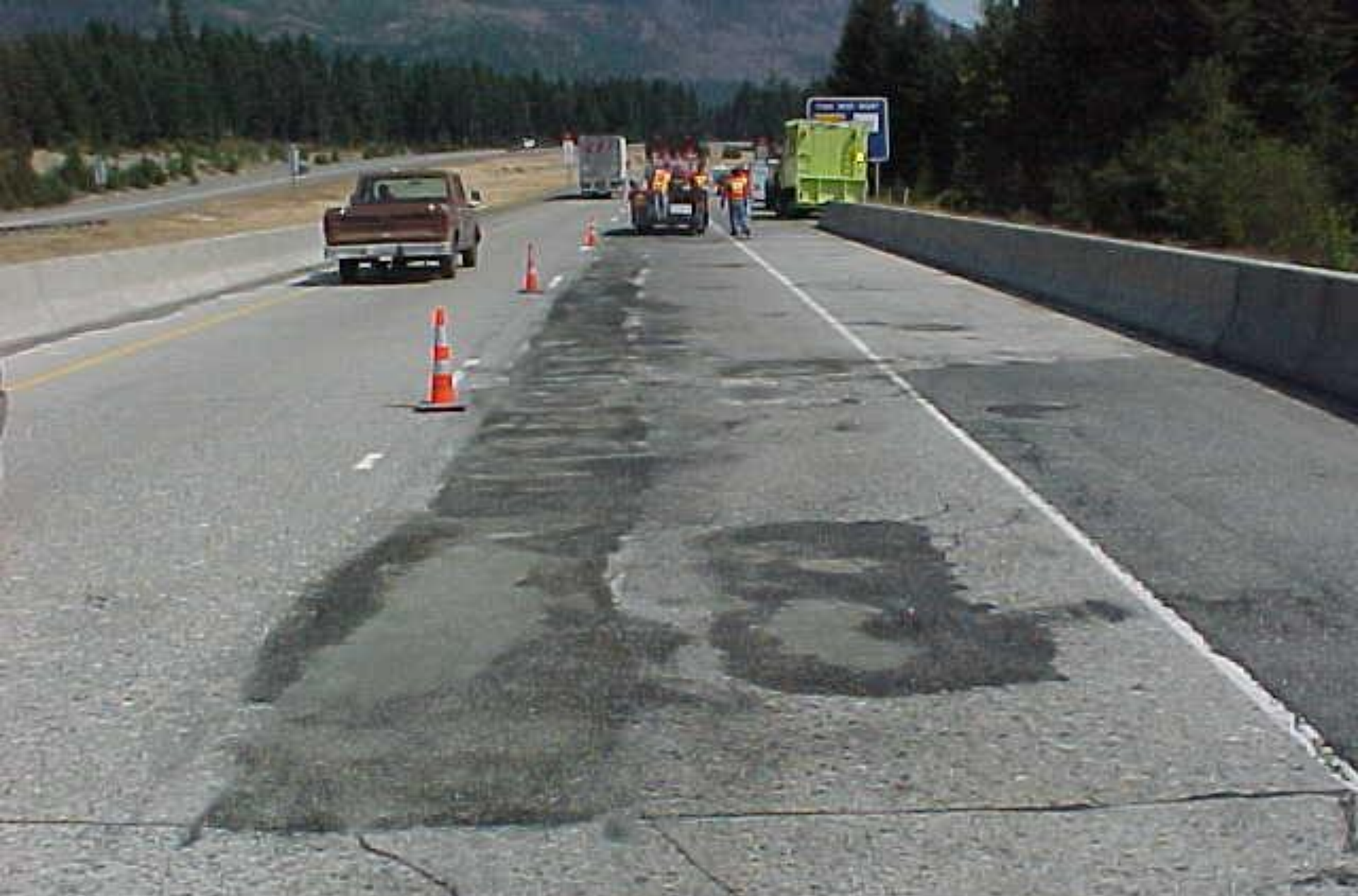
Bridge Deck Repair by WSDOT Maintenance Forces
